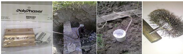
(L - R) Fig 5: This copper-strap clamp secures the strap to the ground rod; Fig. 6: Seven-strand copper wire can be used as a pigtail; Fig. 7: This cad weld is ready to fire; Fig. 8: Use a stainless-steel wire wheel to clean the strap before soldering.
